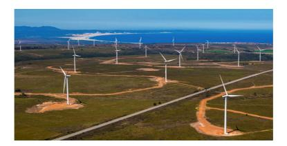
Located between Jeffreys Bay and Humansdorp in the Eastern Cape, the Jeffreys Bay Wind Farm site spans 3700 hectares. The site's optimal wind conditions, relatively flat topography, minimal environmental constraints and its close proximity to the 132kV Eskom grid line, make it an ideal wind energy resource.
